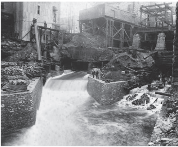
Tailrace construction, about 1900, Minnesota Historical Society
