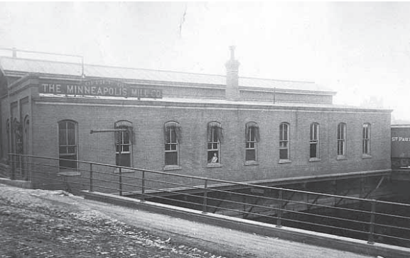
Minneapolis Mill Company Gatehouse, 1895, Minnesota Historical Society
