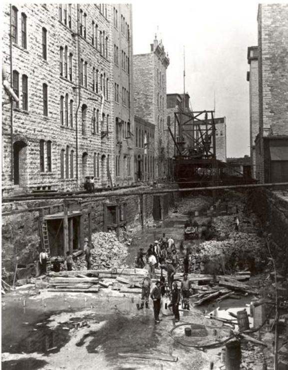
Canal reconstruction, about 1890, Minnesota Historical Society
