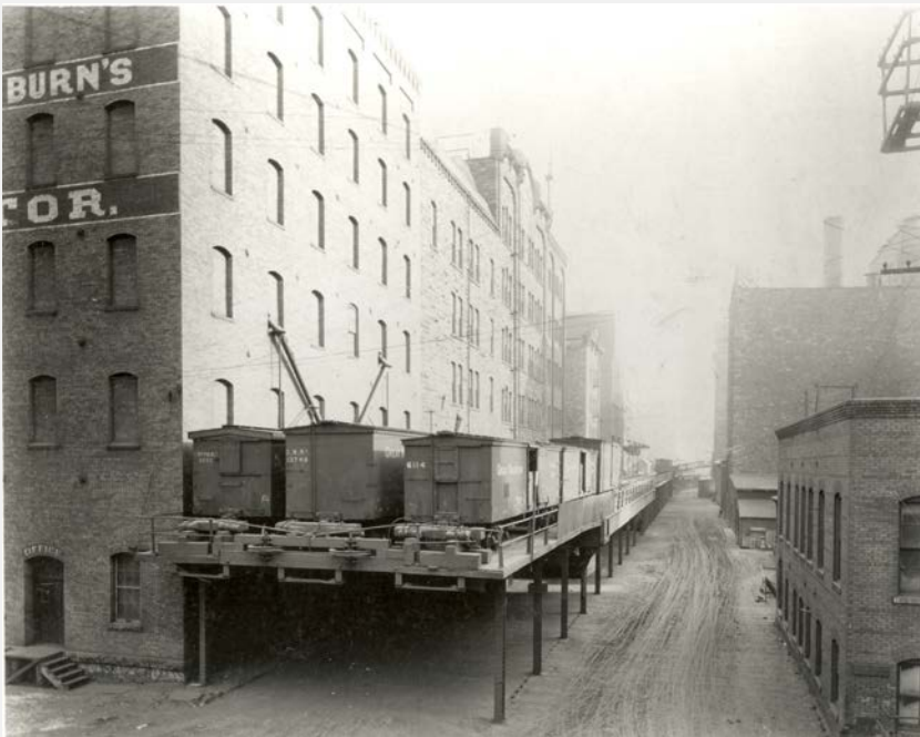
Boxcars were hitched to chains that ran under the tracks, pulling them into position next to the mills then back to engines waiting at the end of the trestle. Photo taken from what is now the corner of Portland Avenue and West River Parkway, river to the left, about 1890. Hennepin History Museum
