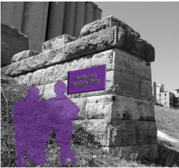
Bridge pier from the Minneapolis Eastern Railroad Trestle.
