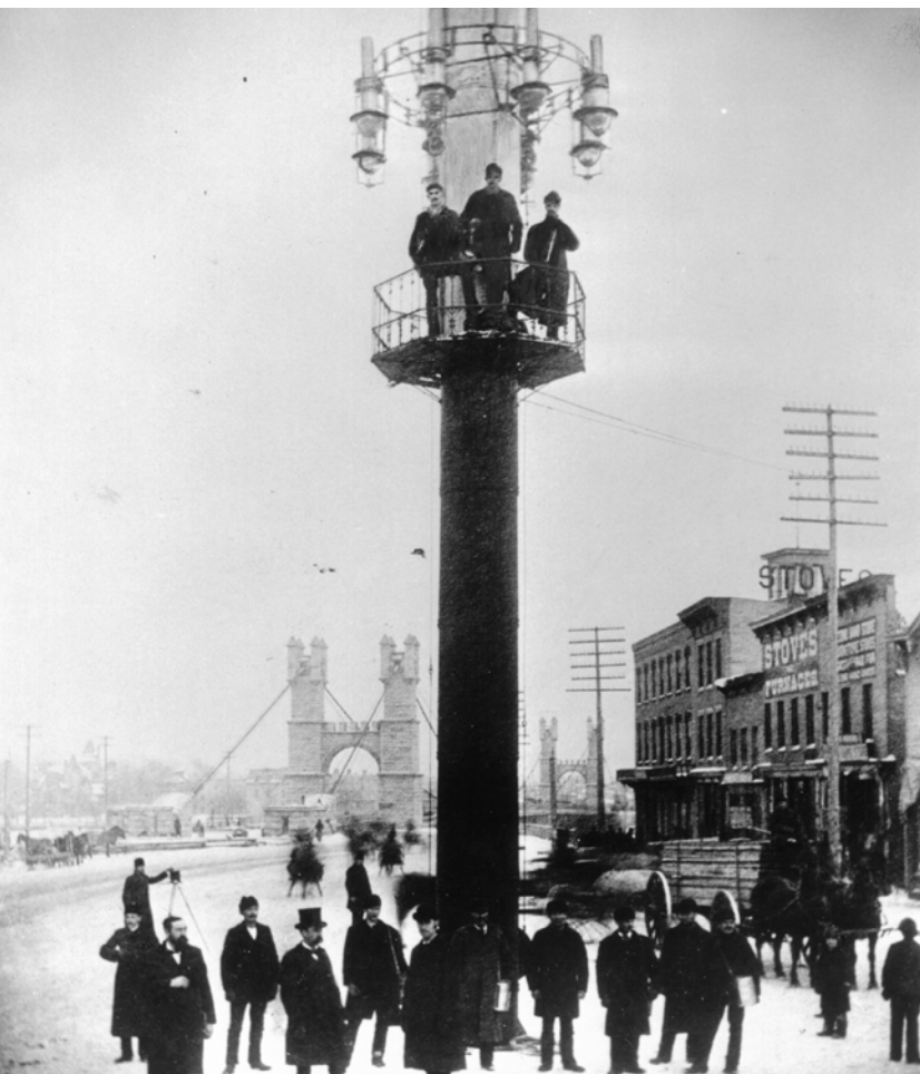
Bridge Square lighting mast, 1883, powered by the Minneapolis Brush Electric Company, Upton Island, the first hydroelectric central station in North America. Minnesota Historical Society
